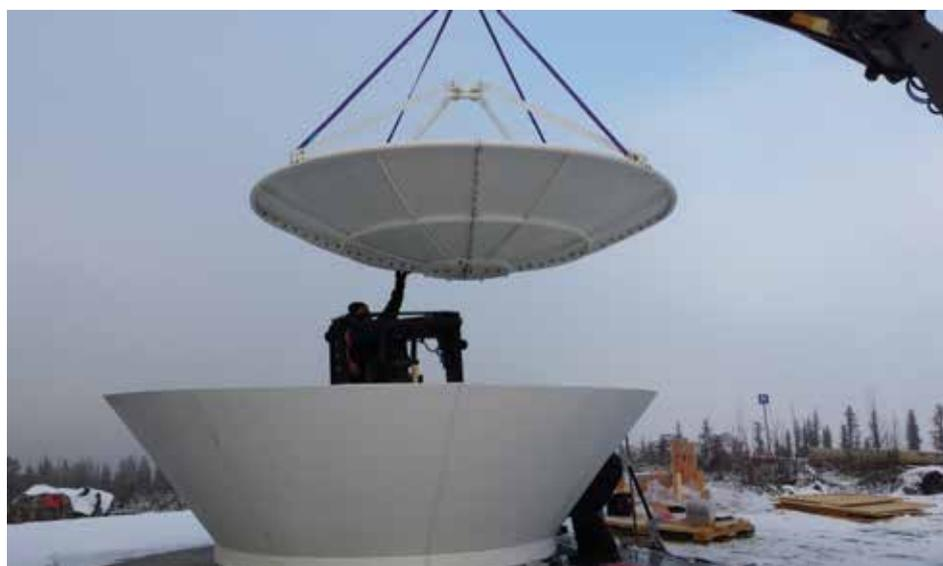
**image 1:** Installation of a smallsat-tracking ground station in a polar environment. **Credit:** courtesy of Orbit Communications Systems, Ltd.
